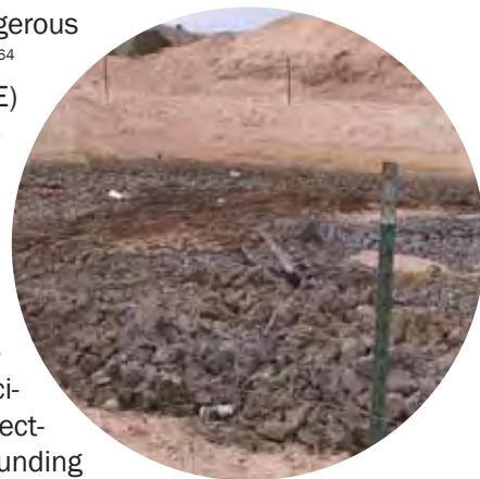
FIGURE I-5. DEWATERED DRILLING MUD Is often buried on-site.
