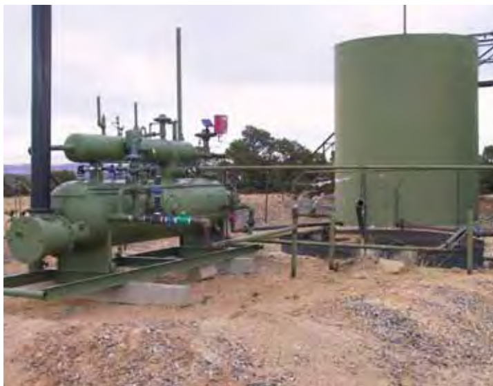
FIGURE I-10. SEPARATOR AND STORAGE TANK FOR THE SEPARATED LIQUIDS
