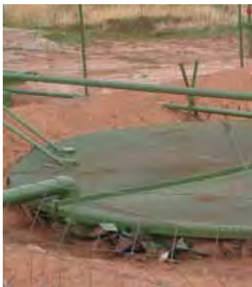
FIGURE I-26. BURIED CONDENSATE TANK
